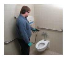
3 Be sure swivel nozzle is set to "S". Start by directing sprayer into toilet and then outside of stool.
